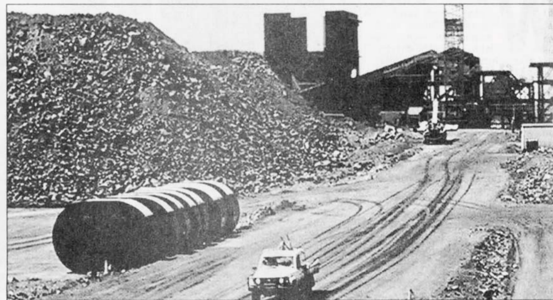
Groundwork: BHP Billiton's Newman mine at Pilbara in Western Australia
