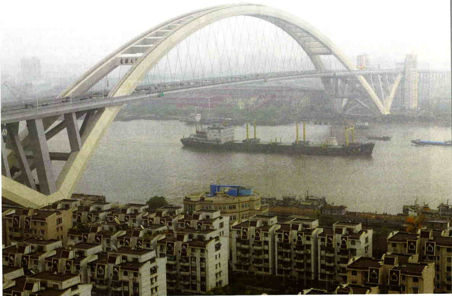
Arcing up: This 550 m long steel-arch bridge across the Huangpu River in Shanghai is the longest of its type in the world. New infrastructure like this is one of the reasons China has become a massive consumer of steel.
